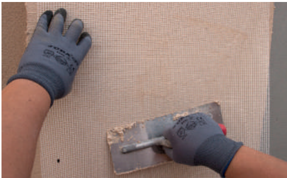
7. Colocar la malla RG-116 Isolxtrem System.
